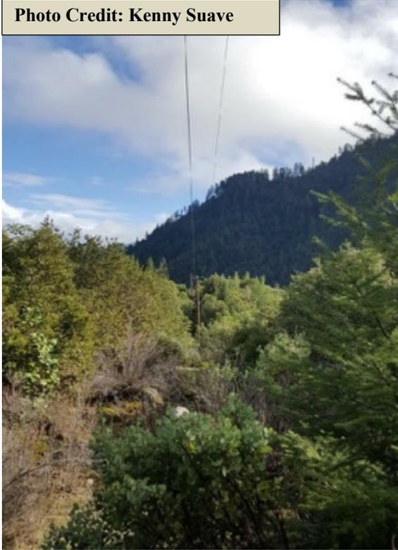
*Figure 5.3 Even Maintained Corridors Have Unsafe Levels of Fuels Near Lines*
